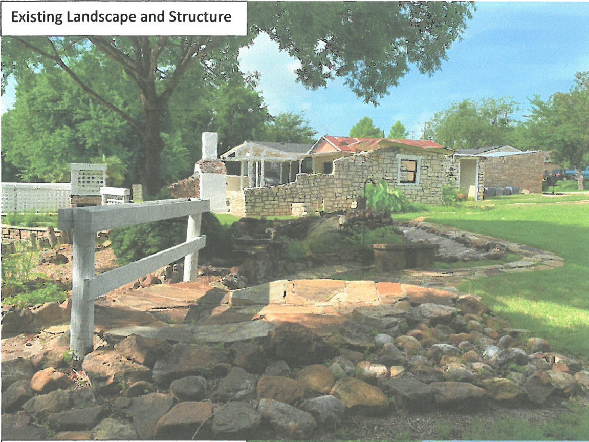
Existing Landscape and Structure
