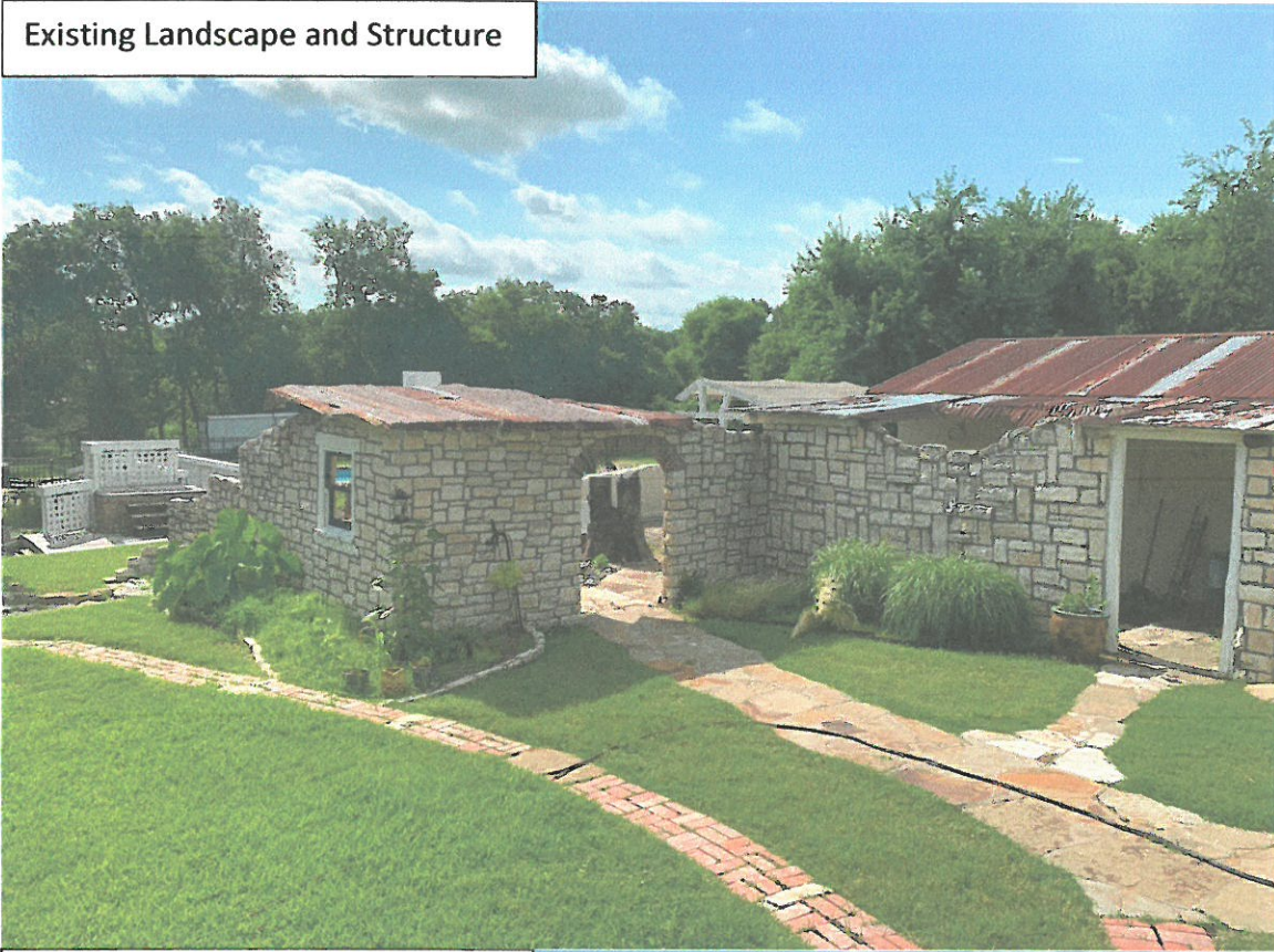
Existing Landscape and Structure
