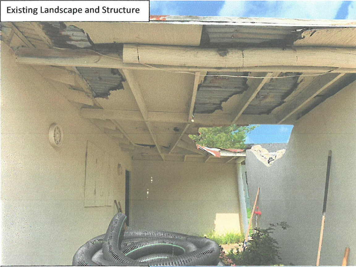
Existing Landscape and Structure
